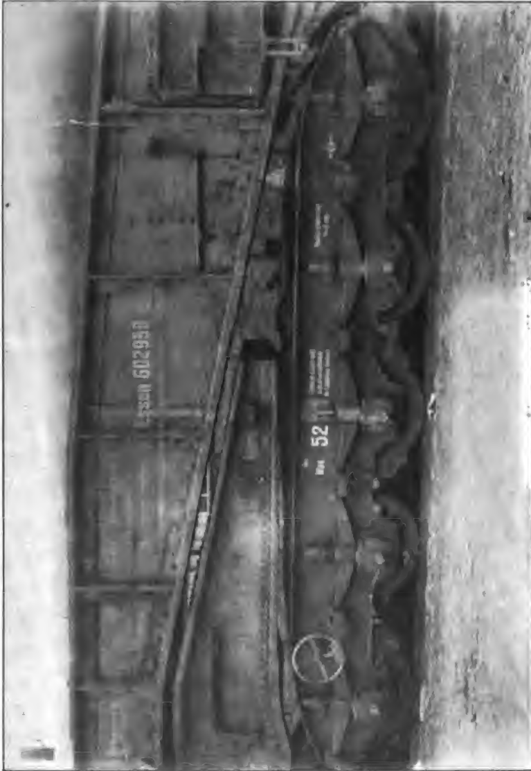
FRONT TRUCK OF 380-MM. GERMAN GUN MOUNT.
